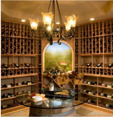
Wine Guardian Ducted Installation. Courtesy: Lakeshore Wine Cellars
