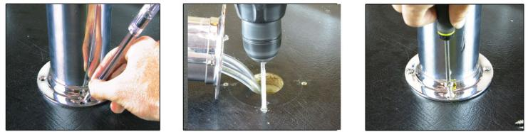
When attaching the faucet to the tower, line up the teeth on the inside of the faucet with the teeth inside the shank. Then screw the coupling nut onto the faucet and tighten with the faucet wrench.
