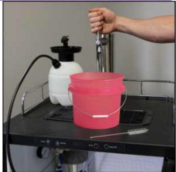
Unlock the pump handle by pushing down and turning the handle. Pump to pressurize the Cleaning Bottle. Place a bucket or pitcher under the faucet and open the faucet to allow the cleaning solution to flow through the line. Pump until dry. Rinse the Cleaning Bottle and fill it with clean, cool water and repeat the cleaning cycle to rinse the line of cleaning chemicals.
